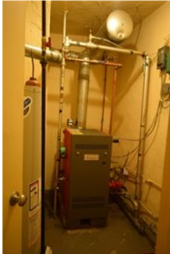
(L-R), Fig. 1: The gas boiler, installed in 2019. Fig. 2: Added baseboard radiators in the bathroom.
