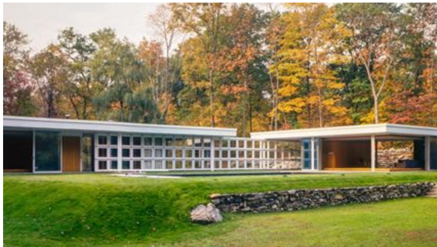
Figure 12: The Morris Greenwald House by Ludwig Mies van der Rohe in Weston, Connecticut (1955).
