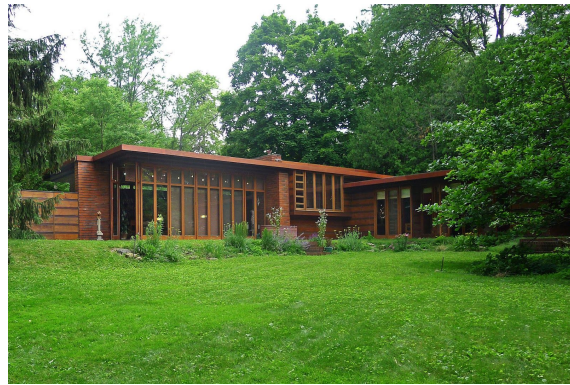
Figure 2. Image showing the rear elevation of the Jacob's Residence
