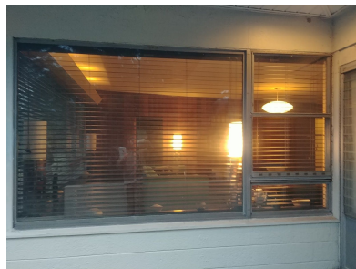
Fig. 4.17 Both operable and inoperable windows.
