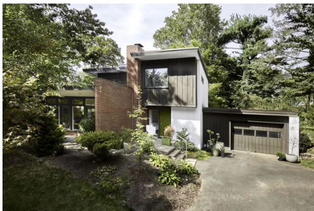
Figure 10. Front of the Berenstain Residence designed by Rice in 1940
