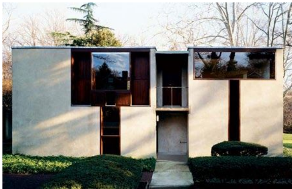
Figure 7. Front elevation of the Esherick home designed by Louis Kahn in 1959
