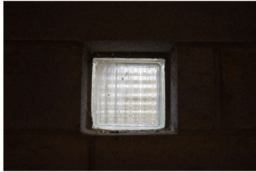
Fig. 4.19 Showing Glass Block in garage.
