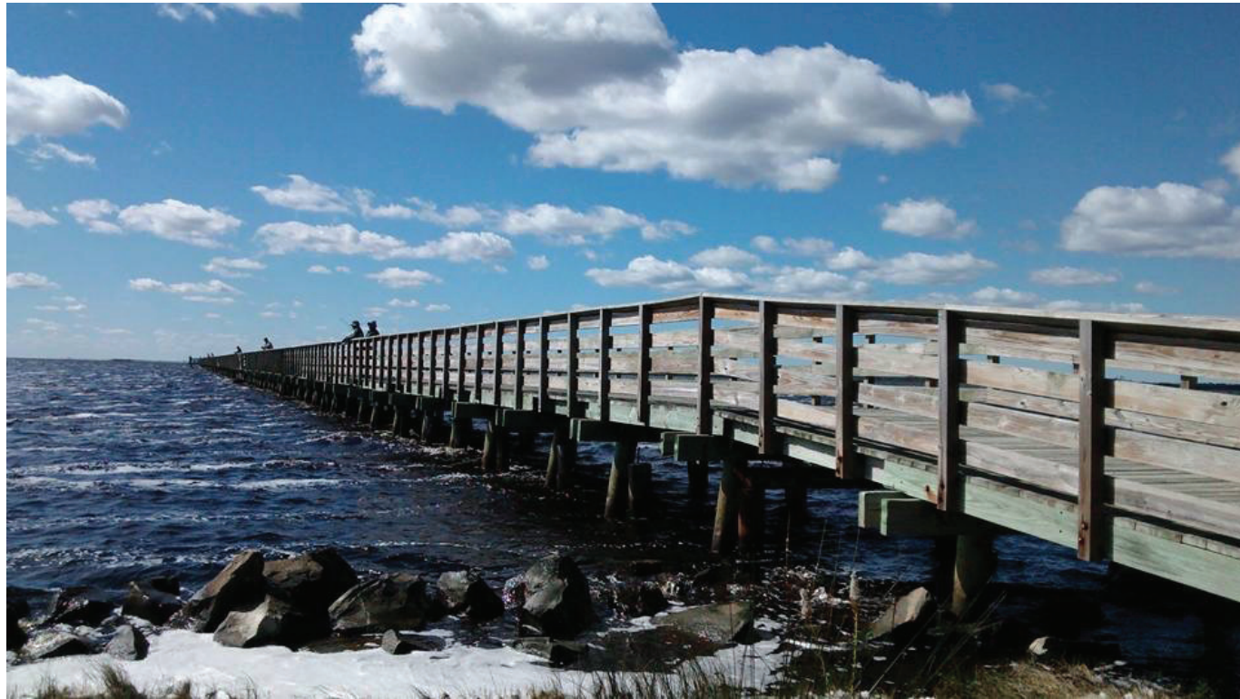
Connections Across the Deep Beverly Anaele Photograph
