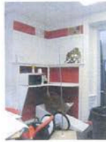
9 Existing Shelving AD2.1
