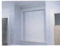
5 Existing Board Against Window AD2.1
